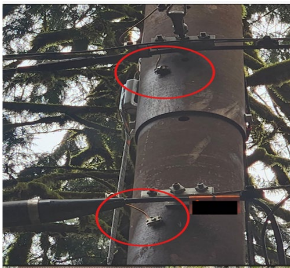
Figure 18. Equipment Grounding Details
