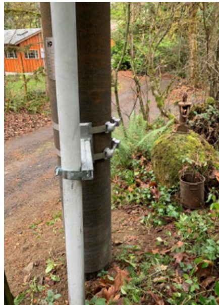
Figure 15. Standoff Bracket Hardware/Banding
