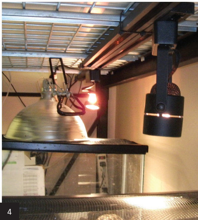
A track lighting system that uses MR-16 bulbs and associated light fixture.
