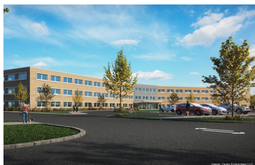
One of PACE Equity's projects is repurposing two former NASA buildings near Cleveland, Ohio, one into energy efficient apartments and the second into an energy efficient hotel. PACE Equity is financing upgrades to the building's envelope, plumbing, insulation, and thermal moisture protection.
