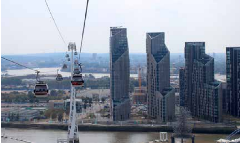
Figure 1.3: Emirates Air Line cable car, looking towards Greenwich Peninsula. Photograph by Hannah Lindner.
