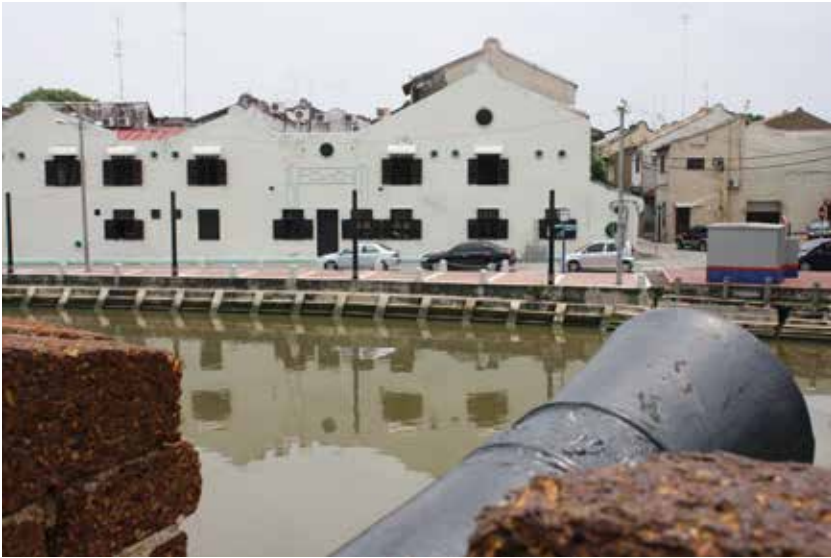
Figure E A view of historical shophouses and townhouses from Bastion Middleburg
