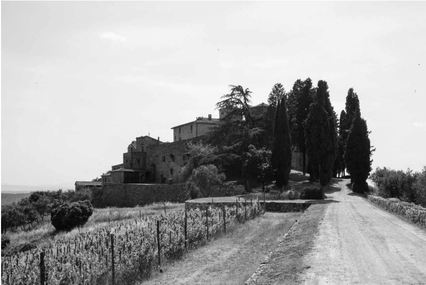
Figure 4: A photograph of the current location of the villa of Cacchiano in Tuscany, which was the country residence of one branch of the Ricasoli family in the sixteenth and early seventeenth centuries. Cacchiano is located in the municipality of Gaioli in Chianti in the province of Siena today, though it was considered part of Florentine territory in the Grand Duchy of Tuscany in the sixteenth and early seventeenth centuries.
