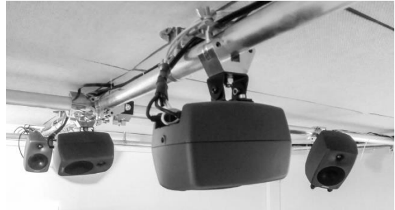
Figure 1a. Method of suspending the upper layer monitors.
