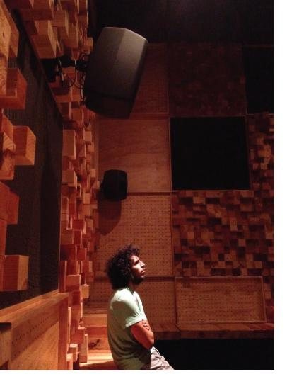
distributor in Latin America, the system generates an immersive sound experience in which where a diversity of moving sounds is reproduced. The whole speaker system is installed within the room which has been acoustically optimized to allow the visitor to focus exclusively on the audio.
