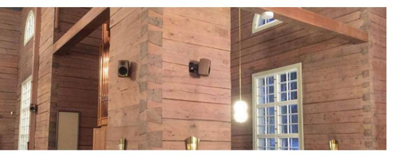
A particular feature of the system tuning for this installation was that we assigned delay to each individual loudspeaker to localize the voice to the person speaking rather than to the nearest loudspeaker using very similar principles and techniques to those used in theatre." The other reason for selecting the 8430A monitors was thanks to their unique IP system distribution qualities. "The clue is in the name!" said Pöykiö with a smile.
