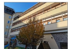
MI – Via Bordoni 2 Office and Kindergarten NRA: 2.500 sqm
