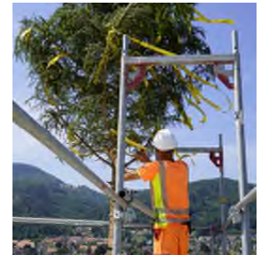
2022 Topping-out of new logistic centre
