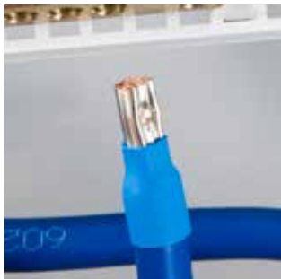
Ferruled cable ends, offer more secure connections
