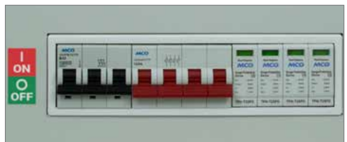
4 Pole 125A Switch Disconnecter, c/w 4 Pole SPD with MCB [supplied]
