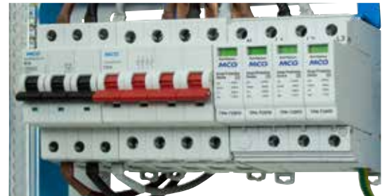
125A Incomer complete with pre-wired T2 SPD and protective MCB
