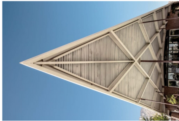
The sweeping roof of the Palm Springs Visitor Information Center, designed by Albert Frey, is known as a hyperbolic paraboloid.
