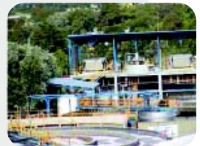
Apizaco Plant, Mexico
