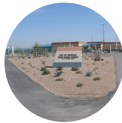
City of Glendale Solar/Storage Development & DER Impact Study
