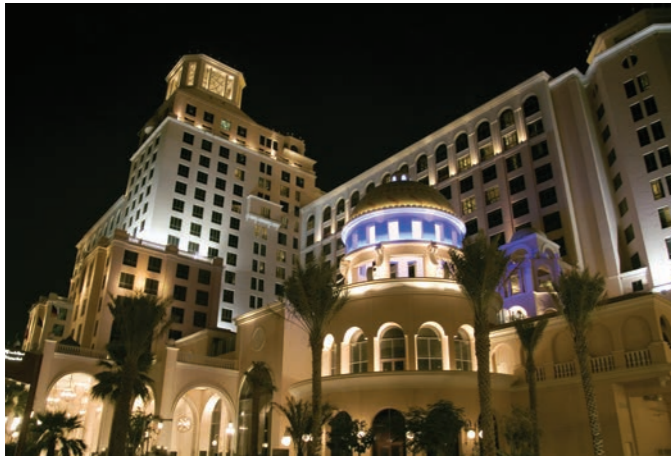
Kempinski Hotel, Mall of Emirates, Dubai, United Arab Emirates
