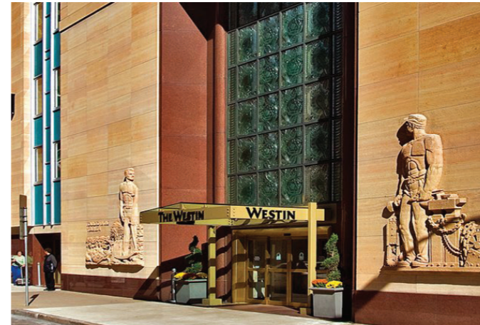
Westin Hotel, Minneapolis, USA
