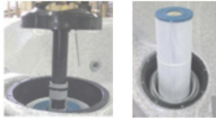
Pull gray tab and turn lock ring counterclockwise. Remove filter lid and cartridge. After cleaning filter, bleed air out of the filter cavity by opening the air relief valve & turn pump on low speed.
