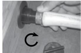
3. Thread hose onto the spa drain
