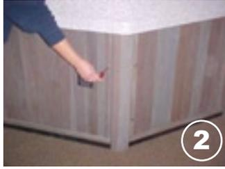
(ST 1056) Install corner posts to side panels using panel bolts and bolt driver.
