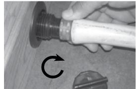
3. Thread hose onto the spa drain
