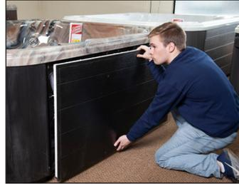
Unscrew and remove the front cabinet panel.
