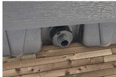
**Step 1:** Remove the drain cap.
