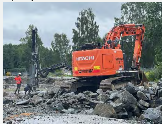
Infrastructure development progressing at Follum.
