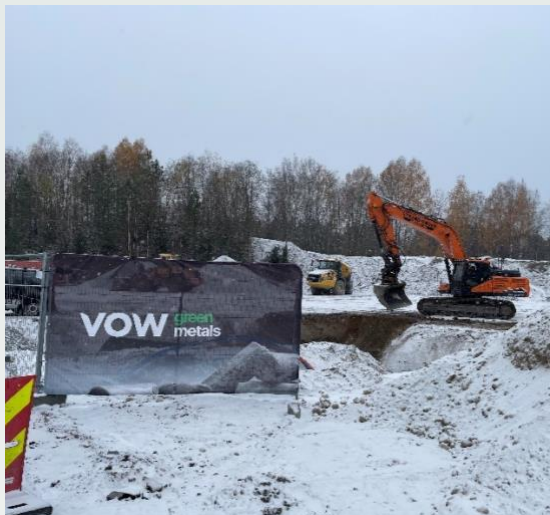
Excavation work conducted by local entrepreneur in October 2023.
