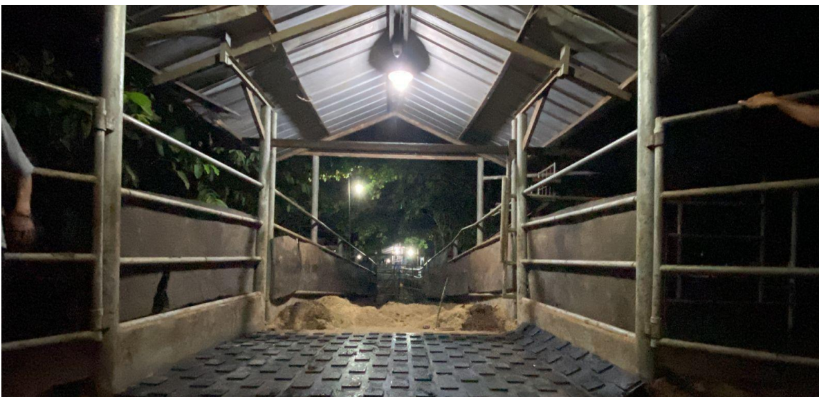
Image: Feedlot unloading ramp with rubber matting installed at the key transition point where cattle step off the truck tailgate onto the ramp.
