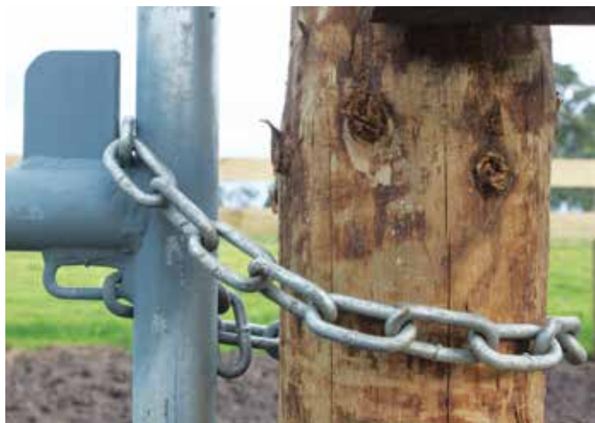
Figure 2.26. Chain latches and spring-loaded 'slam shut' latches are the common closure mechanisms for cattle yard gates. Source: International Agriculture for Development, Commander Ag-Quip.
