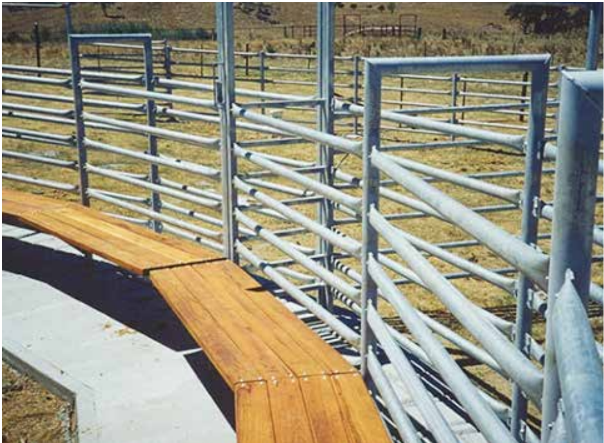
Figure 2.15. Elevated walk platform along the race allows easy access to cattle in the race. Source: Eco Enterac.
