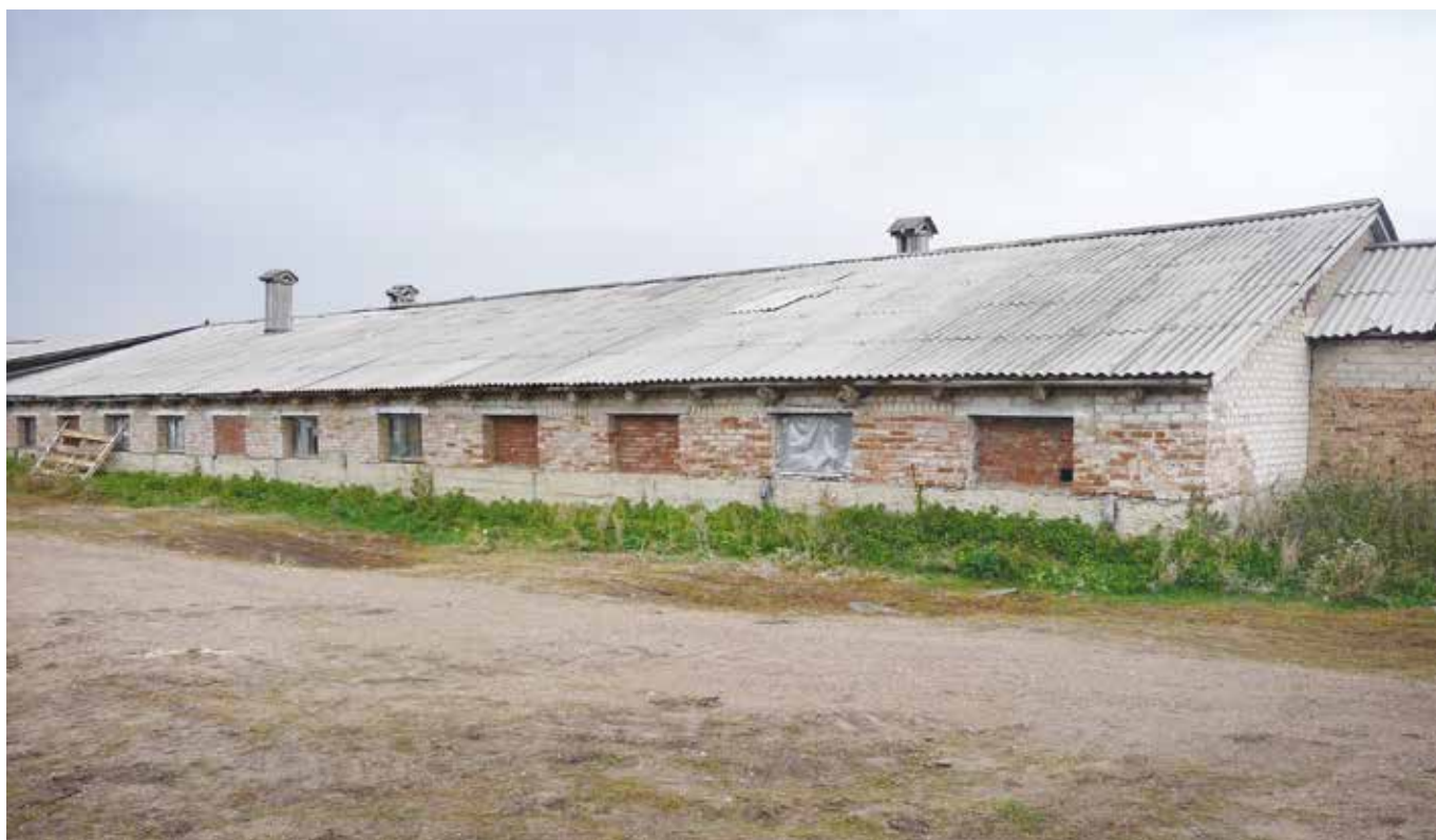
Figure 2.38. Many older sheds have asbestos roofing materials that need to be handled carefully if it is disturbed during a renovation project. Source: International Agriculture for Development.
