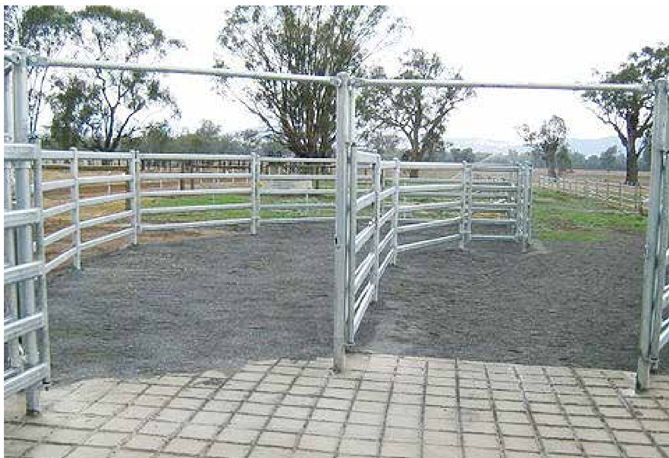
Figure 2.28. Example of cap rails on gates to stop posts from spreading. Source: Proway.
