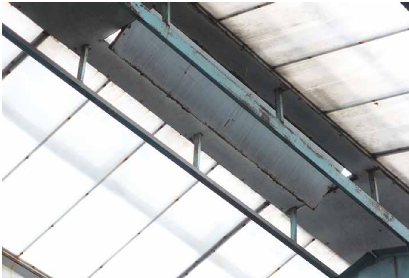
Fig. 2.35. Roof vents improve ventilation and air quality in the shed. Source: International Agriculture for Development.
