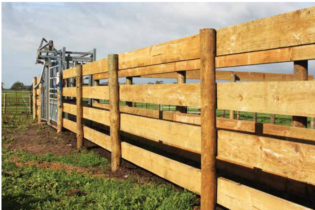
Figure 2.17. Example of wooden rail spacing for cattle yards. With a post height of 1.6m, rails are 200mm wide, and spaced 200mm apart. Source: International Agriculture for Development.
