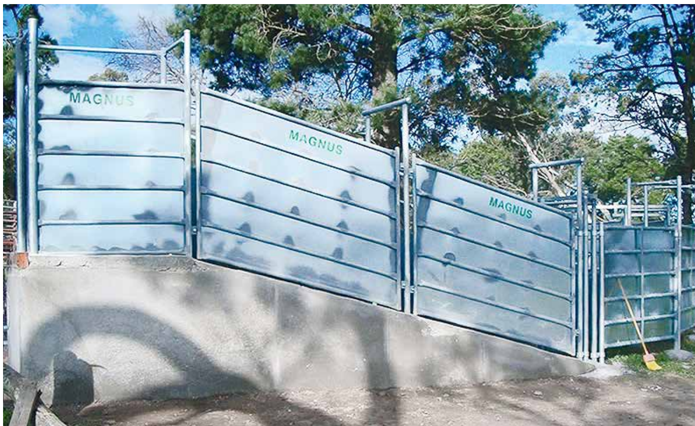
Figure 2.23. Cattle loading ramp with a level platform at the top of the ramp to assist cattle to steady themselves as they step off the truck. Source: Magnus Australia.
