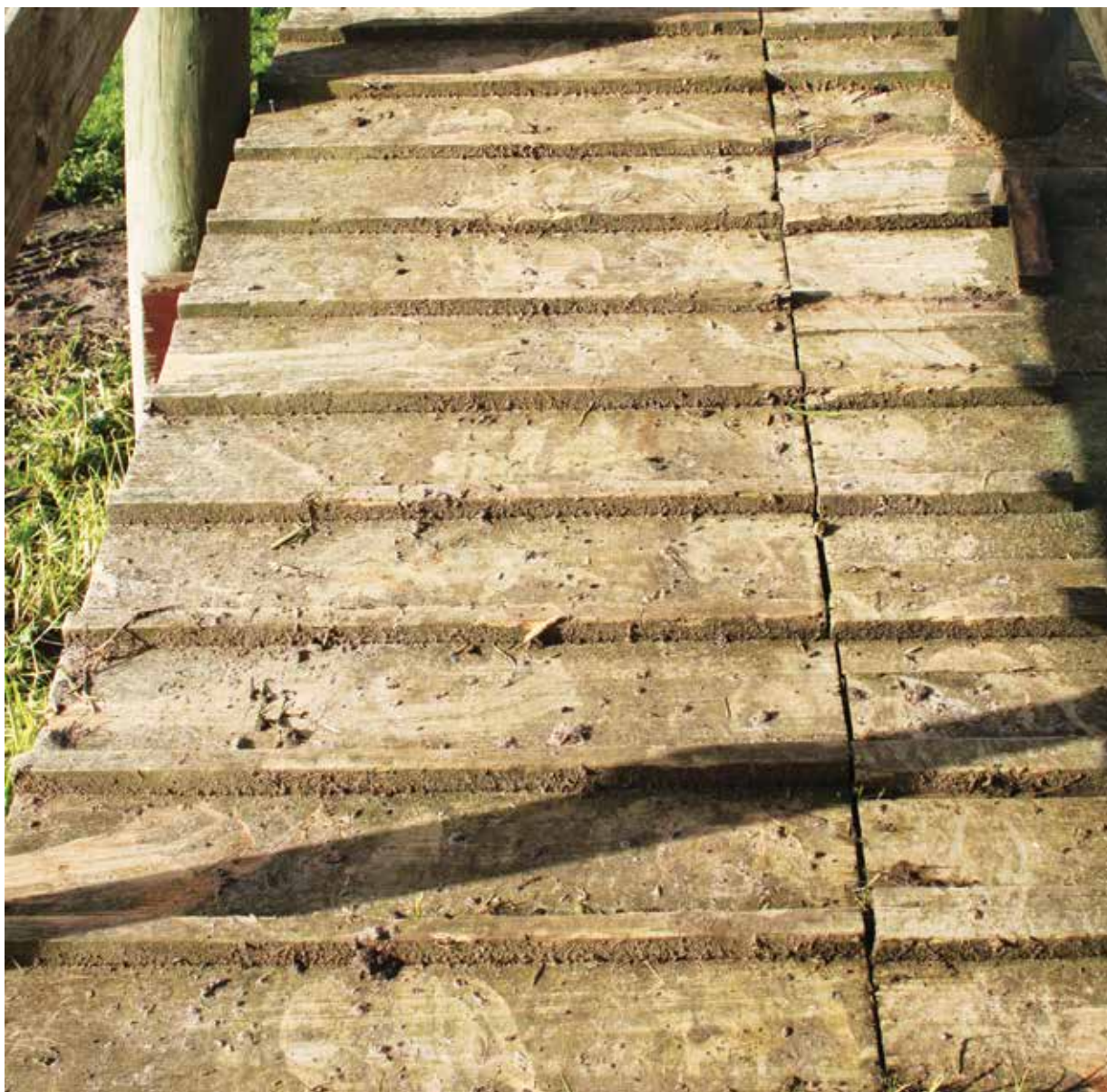
Figure 2.22. A non-slip surface created using narrow tread boards installed across the floor of a wooden loading ramp. Source: International Agriculture for Development.
