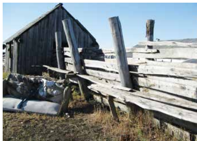
Figure 2.24. Poorly designed and constructed handling facilities such as the flimsy, low-sided loading ramp (left) and poorly maintained race (right) are unsafe for cattle and people and must be replaced. Source: International Agriculture for Development.
