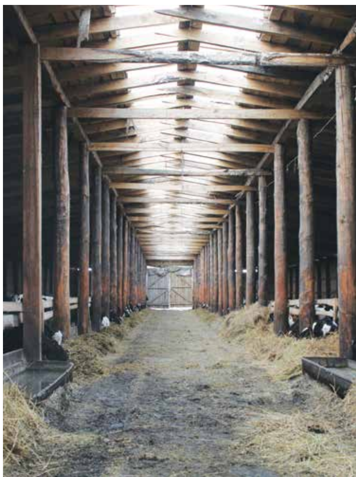
Fig. 2.35. Roof vents improve ventilation and air quality in the shed. Source: International Agriculture for Development.
