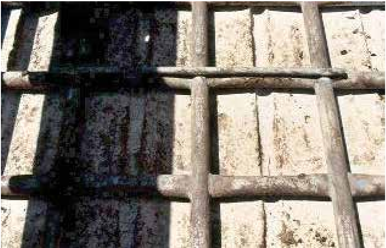
Figure 4.11. Welded pipe cleats provide good footing and reduces slipping, injuries, and deaths. Source: LiveCorp & Meat & Livestock Australia.
