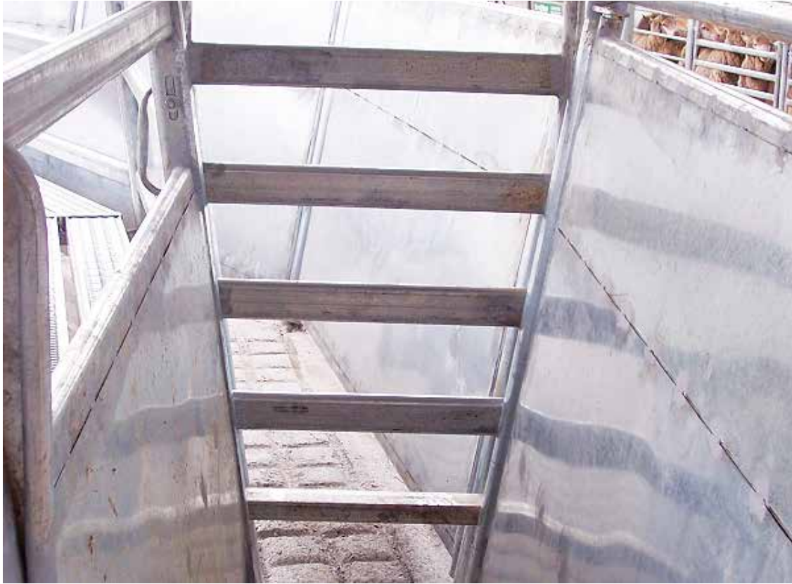
Figure 2.14. Sheeted V race. Note the textured finish to the concrete floor of the race to prevent animals slipping. Source: Proway.
