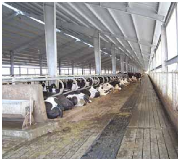
A free-stall barn with side curtains closed to keep the barn warm. The flush alley has a rubber mat running the length of the barn for the cows' comfort and reduced wear on the cows' feet.
