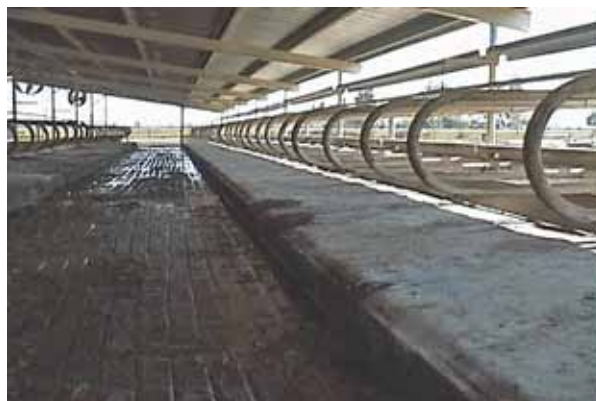
In flush alleys, concrete is grooved in the direction of cow and effluent flow.
