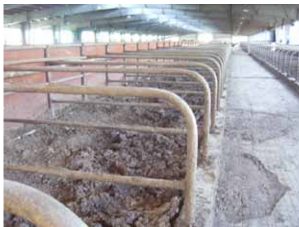
These free-stalls are short and the cows have nowhere to lung forward or to the side when they attempt to stand up. There is insufficient bedding and the bedding that is present is hard. Not surprisingly, all of the cows chose to lie outside in a muddy yard.
