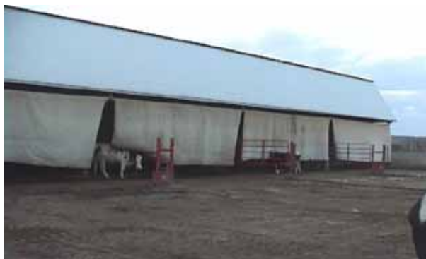
Side curtains are used in sheds in colder climates. They can be raised in summer and lowered in winter.
