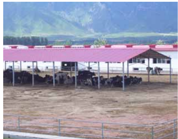
Well-maintained loafing yard with provision of shade. Ideally sunlight should be able to reach all areas under the shade at some point of the day to help keep the surface dry.
