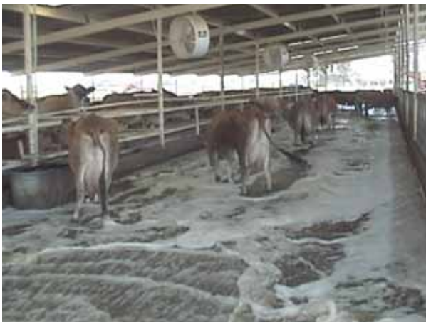
Flush alleys should slope in the direction of the effluent flow with a 3% slope to allow quick and free drainage of effluent.
