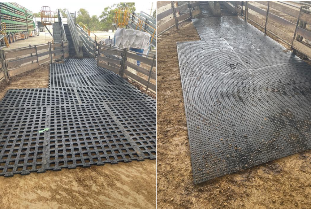
Image: Post installation of interlocking Airstud with custom holes (left) and Airstud with straight edge (right)
