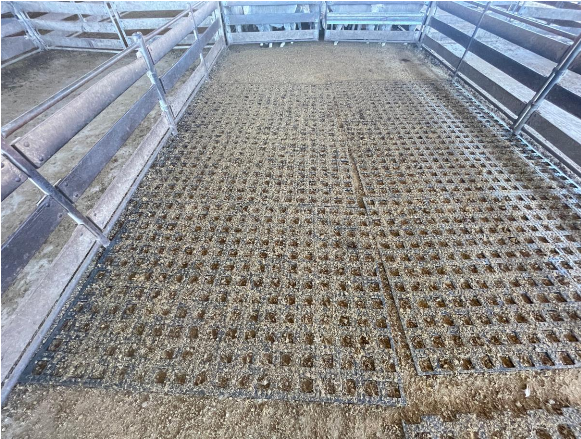
Image: Mats without interlocking edges moved over time due to inability to permanently secure.
