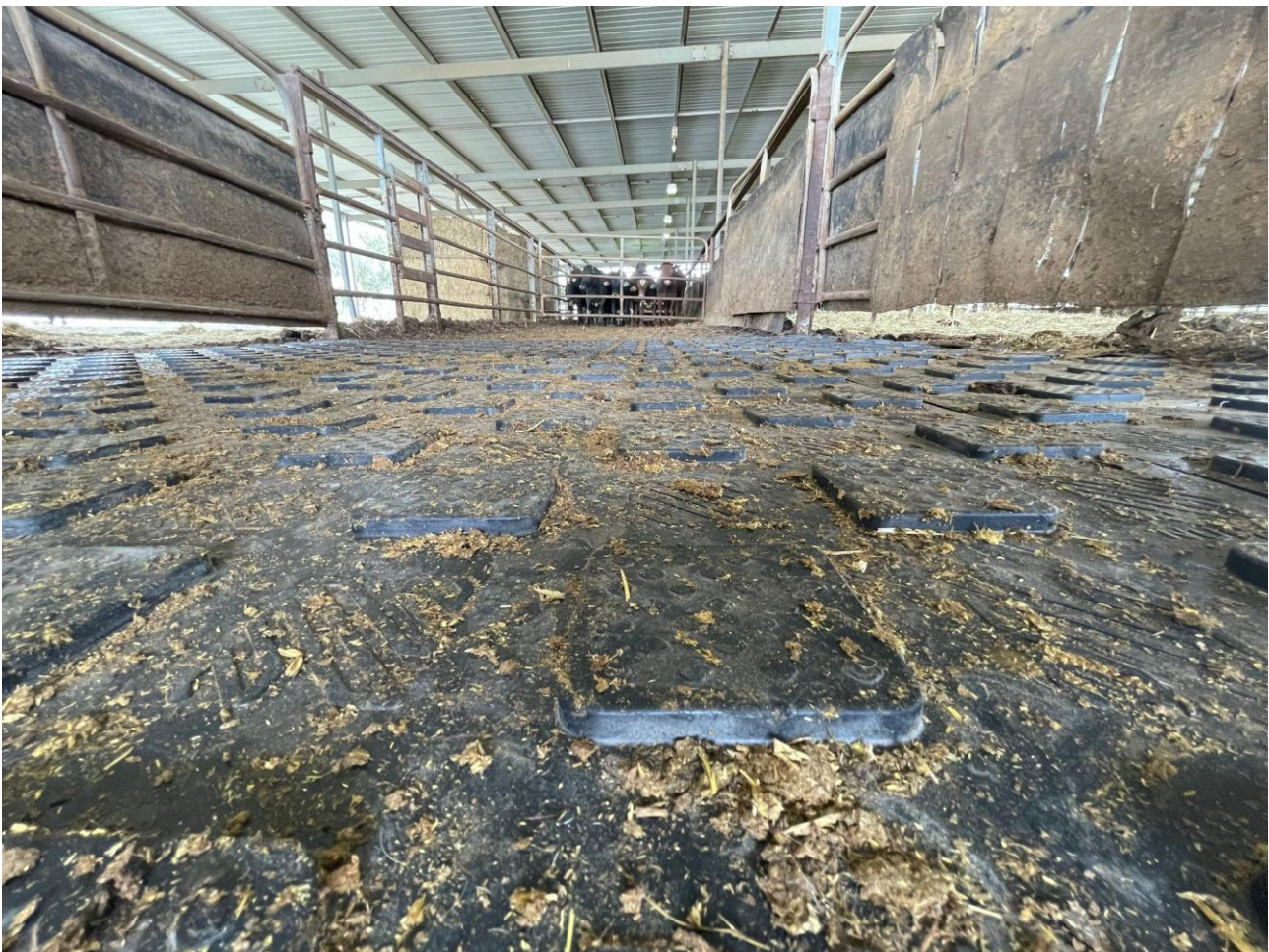
Image: YoungStar mat installed at site 1
