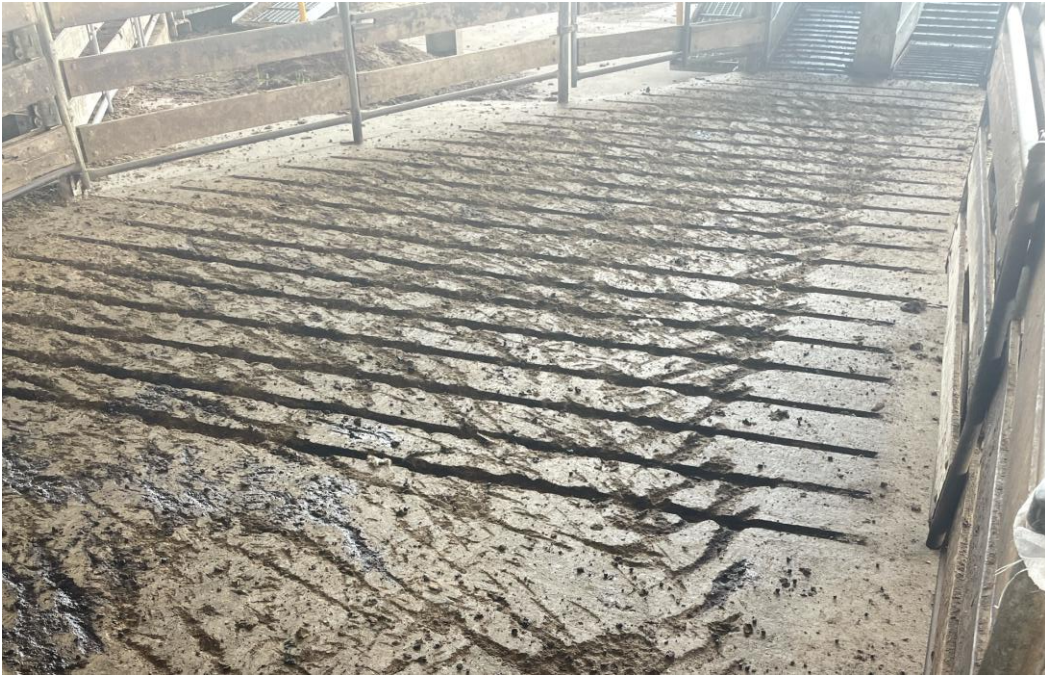
Image: Pre- installation surface at the bottom of the loading ramp.
