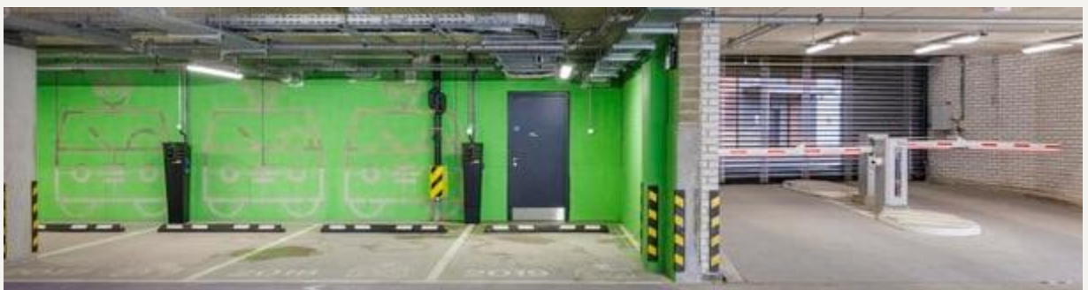
Exhibit 12: ONE Station Hill Parking Garage
