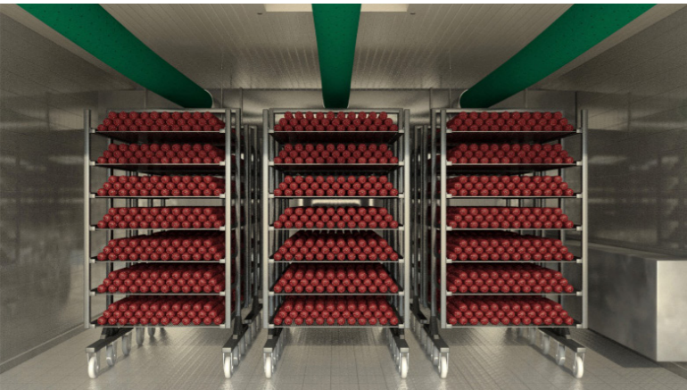
Fig.1 Air distribution with hose system
