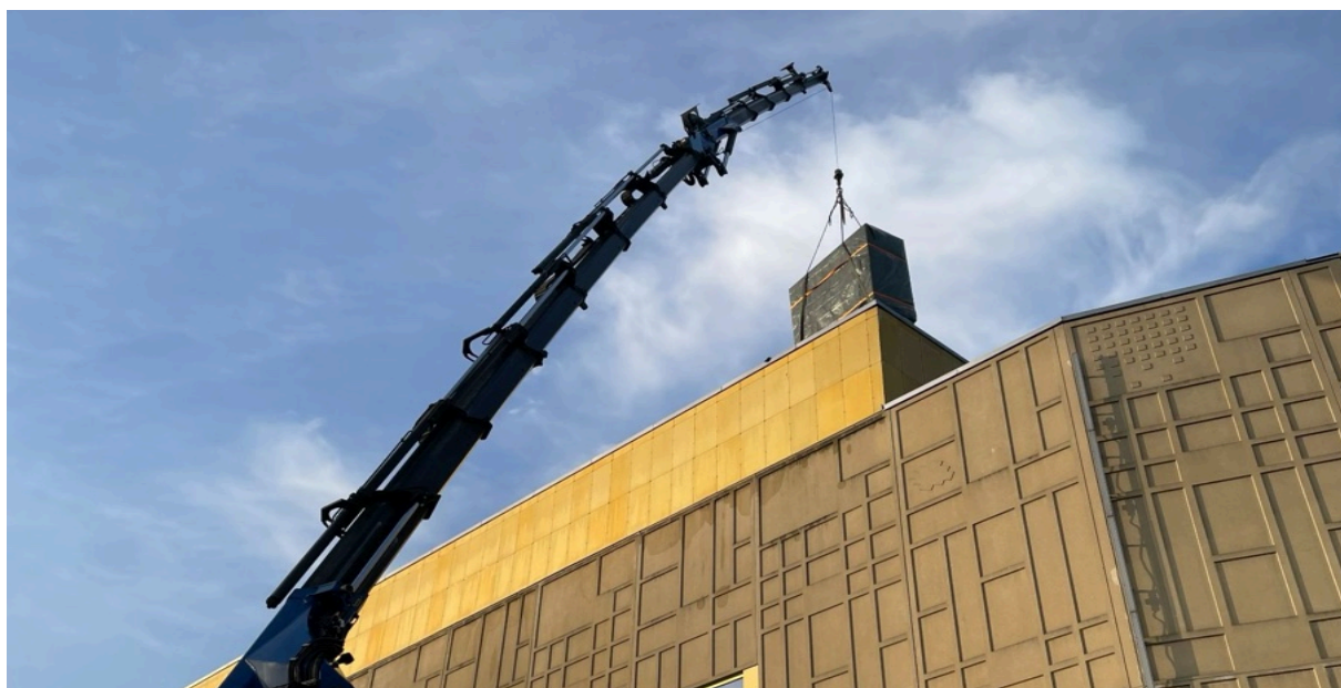
Picture: Dismantling HVAC equipment at Galleria Boulevard by Boulevardfastigheter, Kristianstad, 2026
