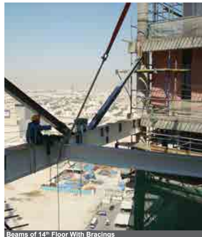
Beams of 14 th Floor With Bracings
