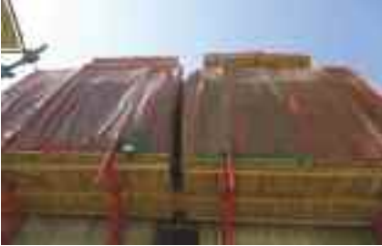
| Core hydraulic system
