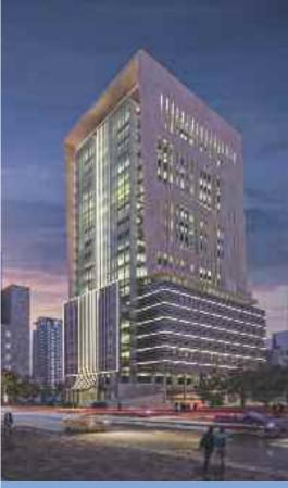
The project consists of the turnkey construction of the office tower comprised of a basement, ground floor, seven upper floors serving as parking spaces, and 13 floors of office space.
