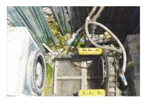
This process avoids the need to have long stretches of open trench for pipe laying, which causes extreme disruption, especially in a congested residential area. This can be particularly important when trying to install a new pipeline in an area where a maze of underground utility lines already exists.
