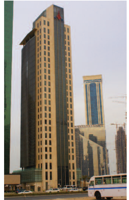
AMWAL TOWER, QATAR CONCRETE WORKS COMPLETED IN 11 MONTHS. SLAB CYCLE REACHED 4 DAYS IN THE TYPICAL FLOORS.
