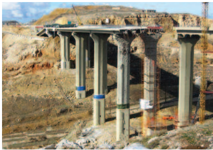
BRIDGE STATUS BEFORE REHABILITATION
