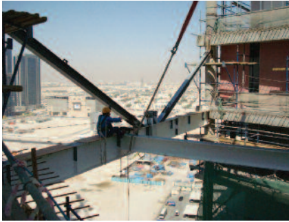
FIGURE 2: BEAMS OF 14 TH FLOOR WITH BRACINGS
