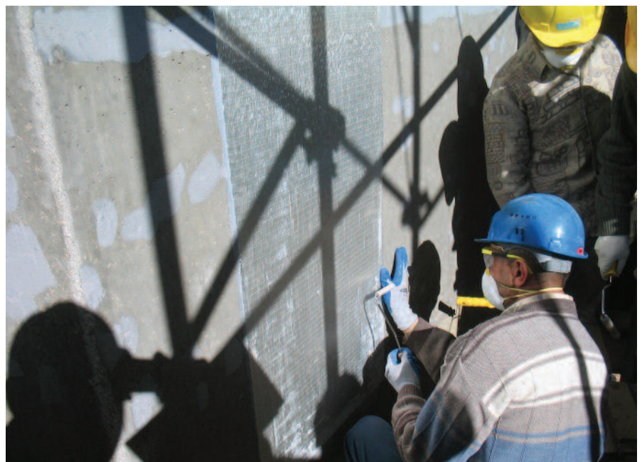
FRP: APPLICATION OF THE FRP
