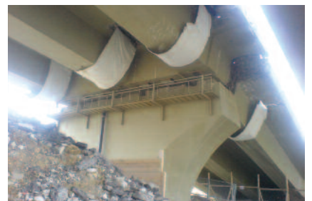
IMPLOSION: EXPLOSIVES SET AND PROTECTED AT DESIGNATED LOCATIONS OF THE BRIDGE
