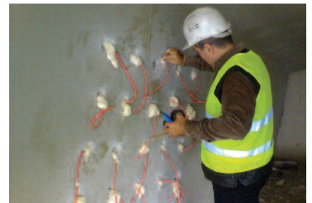
IMPLOSION: IMPLANTATION OF EXPLOSIVES WITHIN A HEAVY DAMAGED PIER
