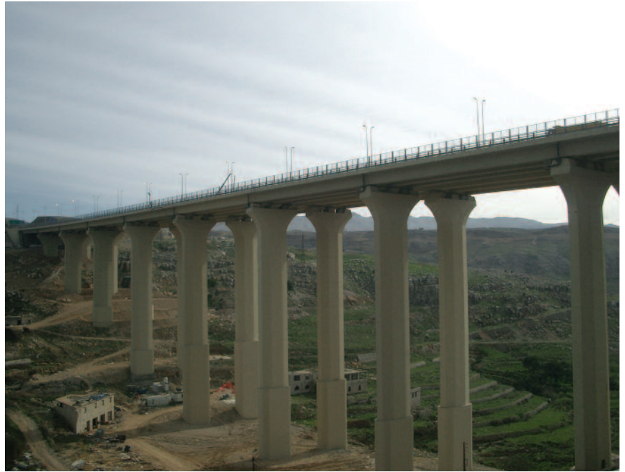
BRIDGE STATUS AFTER REHABILITATION
