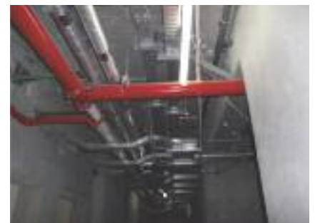
| Electrical Services at Floors Lobby (Cable Trav, EMT) |
