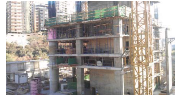
| Photo 3: Insulated massive columns at Crédit Libanais project
