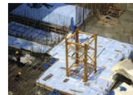
| Photo 2: Insulated mat foundation at the Sky-Gate project.
