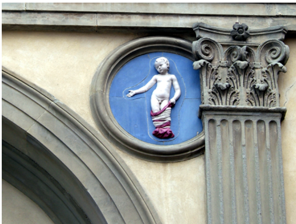
Fig. 6. The Spedale degli Innocenti (Florence) realized by Brunelleschi (1419–1445): a particular element of the façade with its white plaster finishing contrasting with the greyness of Pietra Serena. The façade is adorned with white and blue glazed terracotta tondi depicting babies in arms, works of Andrea della Robbia, added in 1487.
