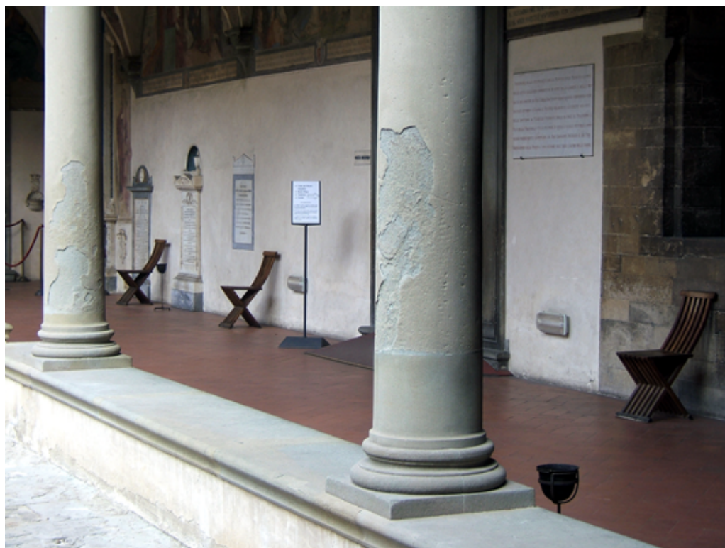
Fig. 13. Decay of Pietra Serena along the columns of the cloister of San Marco Convent (15th century, Florence): the process develops mainly through exfoliation and detachment of crusts.
