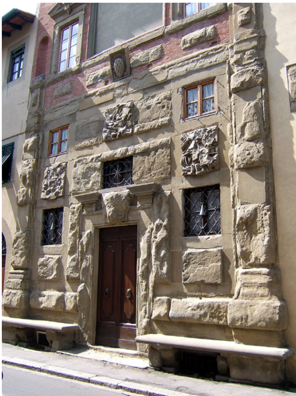
Fig. 8. Architectural element in Pietra Bigia (Zuccari Palace-Florence 16th century), a variety of Pietra Serena which underwent an oxidizing process, which nevertheless did not affect the durability.
