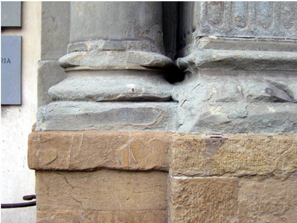
Fig. 2. The two types of sandstone in Florence: Pietraforte at the bottom, rich in convolute laminations and calcite veins; Pietra Serena on top. Pietraforte is the building material of the city while Pietra Serena is mainly employed as ornaments and architectonic decorations.
