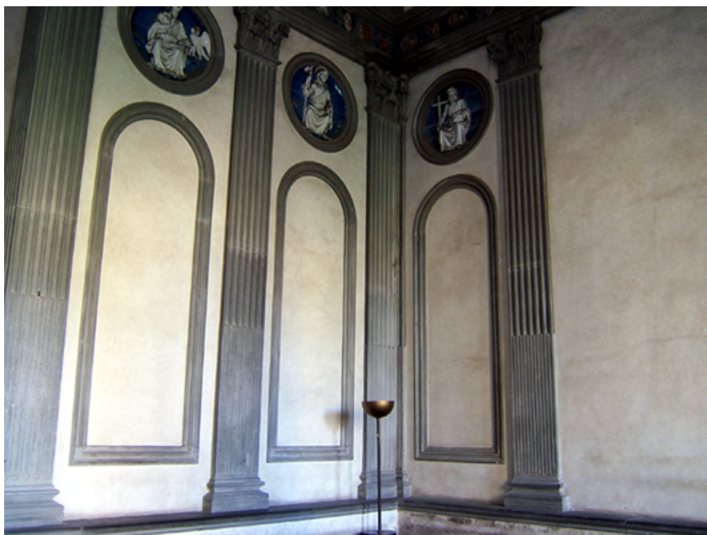
Fig. 5. The Pazzi Chapel within the Franciscan Convent of Santa Croce (Florence), one of the most extraordinary examples of the Renaissance architecture, which construction was initiated by Brunelleschi in 1429. It is evident that the white plaster finishing contrasts with the grey of the Pietra Serena architectural elements.
