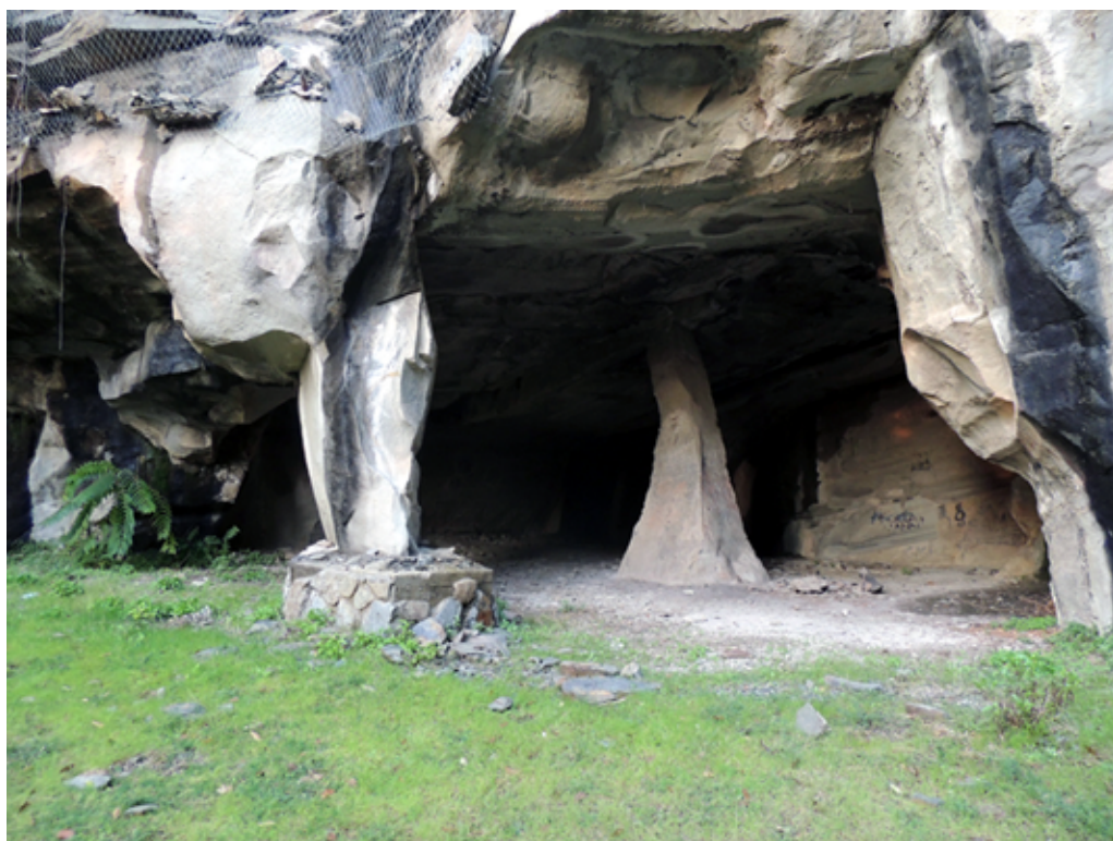
Fig. 9. The Braschi quarry, along the slopes of Monte Ceceri (Fiesole), one of the few quarries where the stone was extracted from the depths of the mountain, which left stone pillars in order to prevent the fall of the vault.
