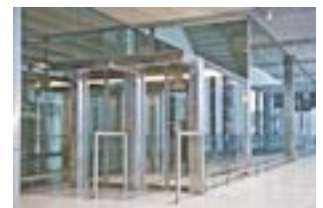
Security doors & barriers
