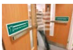
Emergency exit hardware
