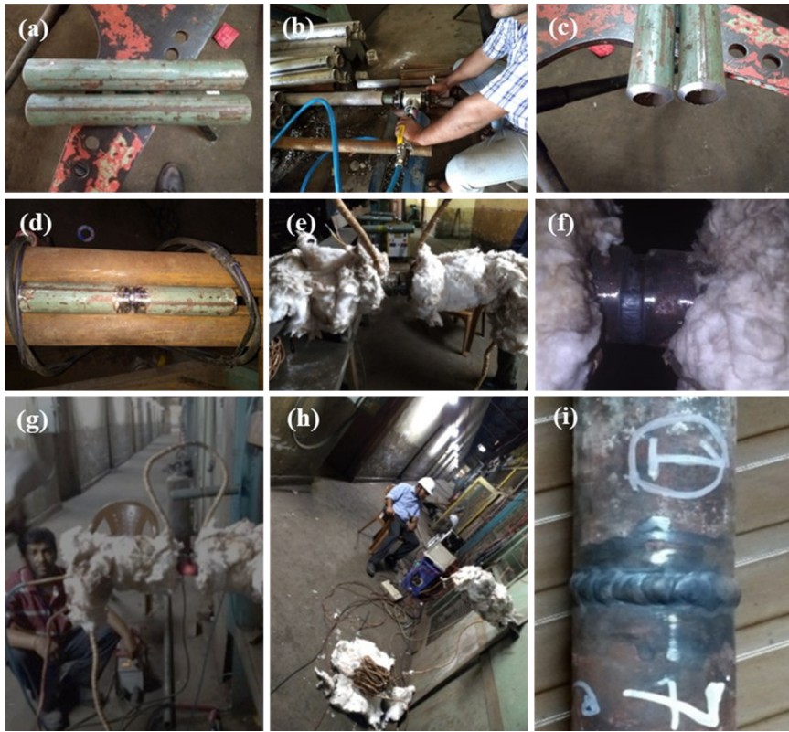
Fig 1. Photographs showing different stages of Welding of T91 Boiler Tubes. (a) Cut to Length, (b) Face or Bevel, (c) Cleaning, (d) Alignment, (e) Root Pass, (f) Hot Pass, (g) Heating Cycle in PWHT, (h) Soaking and Cooling Cycle and (i) Final Welded Tube
