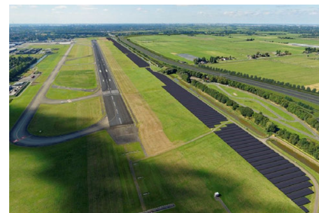
Solar park at Rotterdam The Hague Airport
