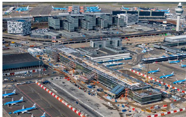
The new A-Pier
