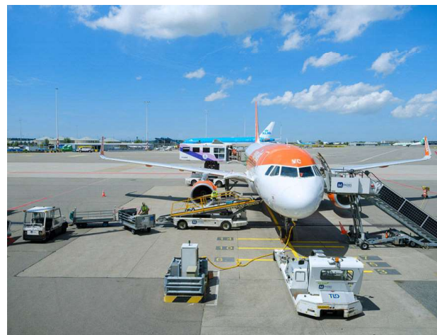
In 2023, maintenance was carried out on numerous aircraft stands in the Pier G, Pier E and Pier D areas. The maintenance project included an element of electrification to support more sustainable airside operations.
