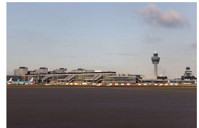
The new Pier A is necessary to guarantee the future demand for new aircraft stands and gates, but also to create redundant capacity to be able to renew or refurbish existing piers.
