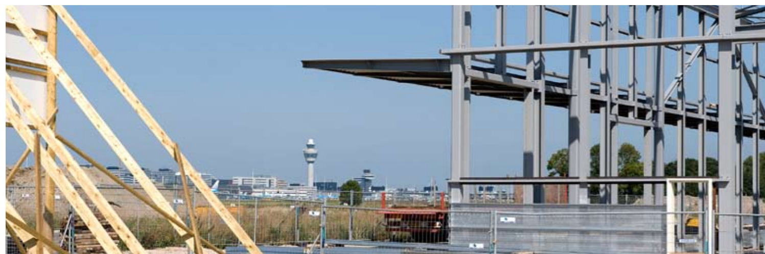
Cargo building for Panalpina under construction at Amsterdam Airport Schiphol
