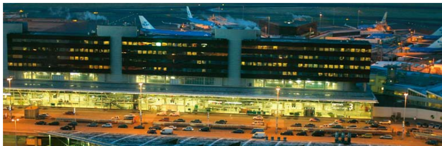
Offices in terminal building of Amsterdam Airport Schiphol
