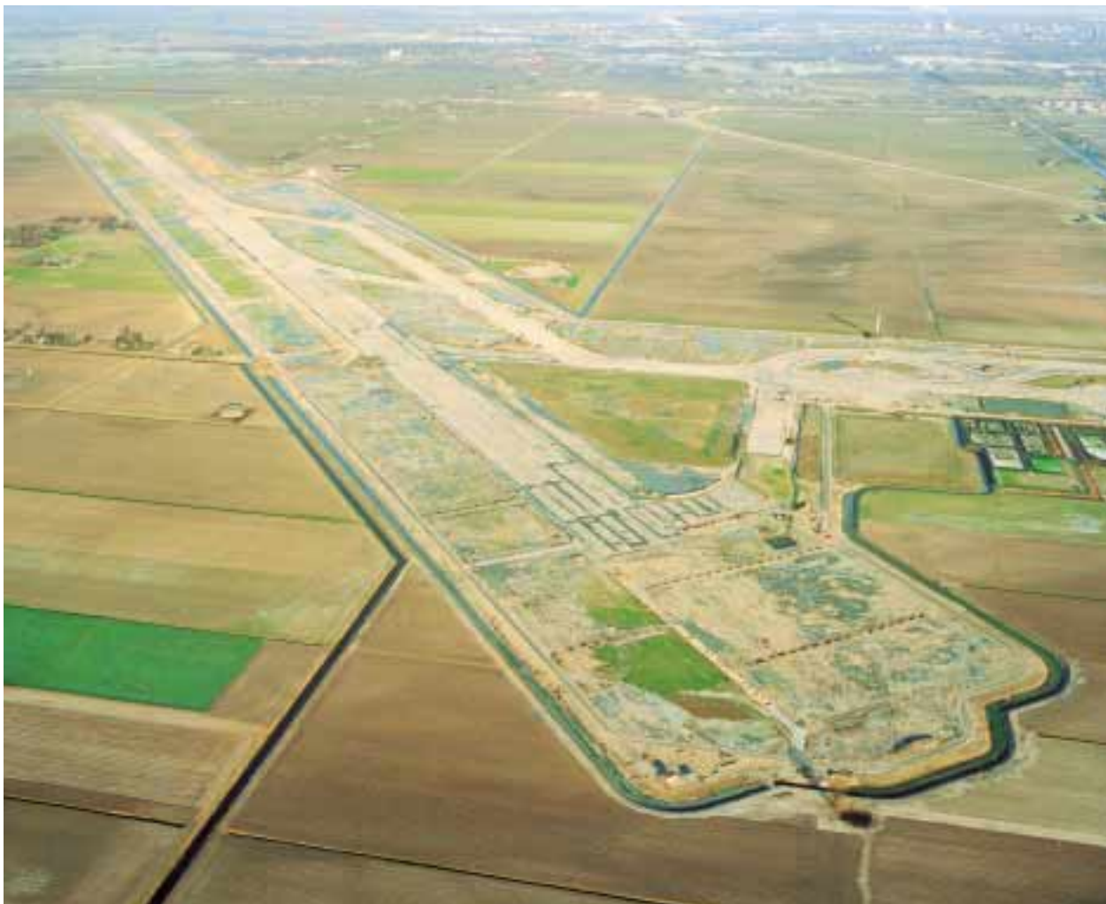
Fifth runway under construction
