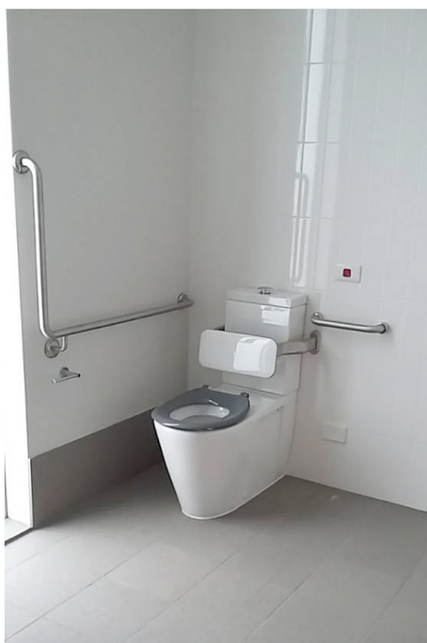
Compliant WC setup, with grabrails
