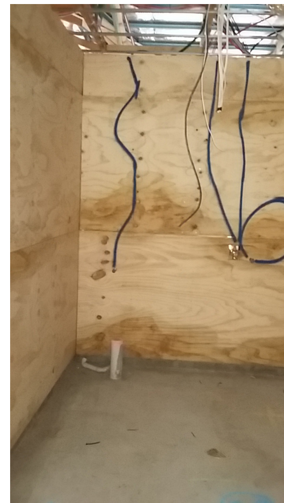
Example of the bathroom plywood-sheeted walls.
