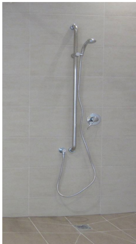
Partially compliant shower – not in corner position, without offsets from wall, shower mixer in corner, or horizontal grab rail
