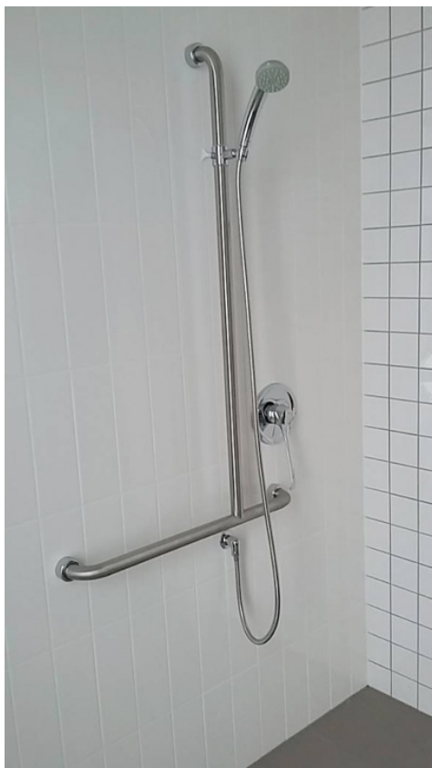
Compliant shower, in corner position with offsets from wall and integrated horizontal grab rail; shower mixer in corner
