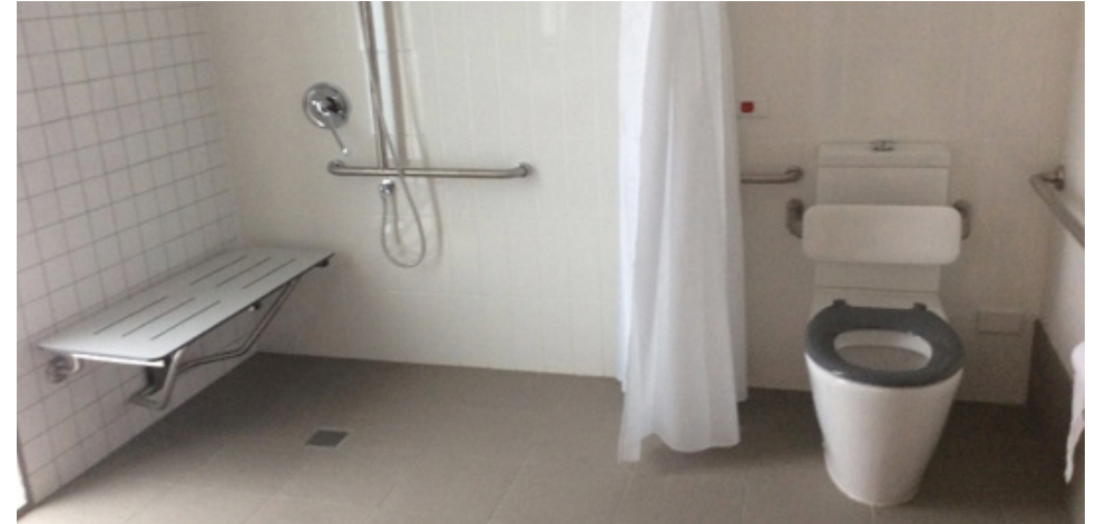
• An example of an 'institutionalised' bathroom compliant to AS 1428.1 within a BCA Class 3 development. Note the requirement for grabrails, shower seat, shower curtain and backrest behind the toilet.
