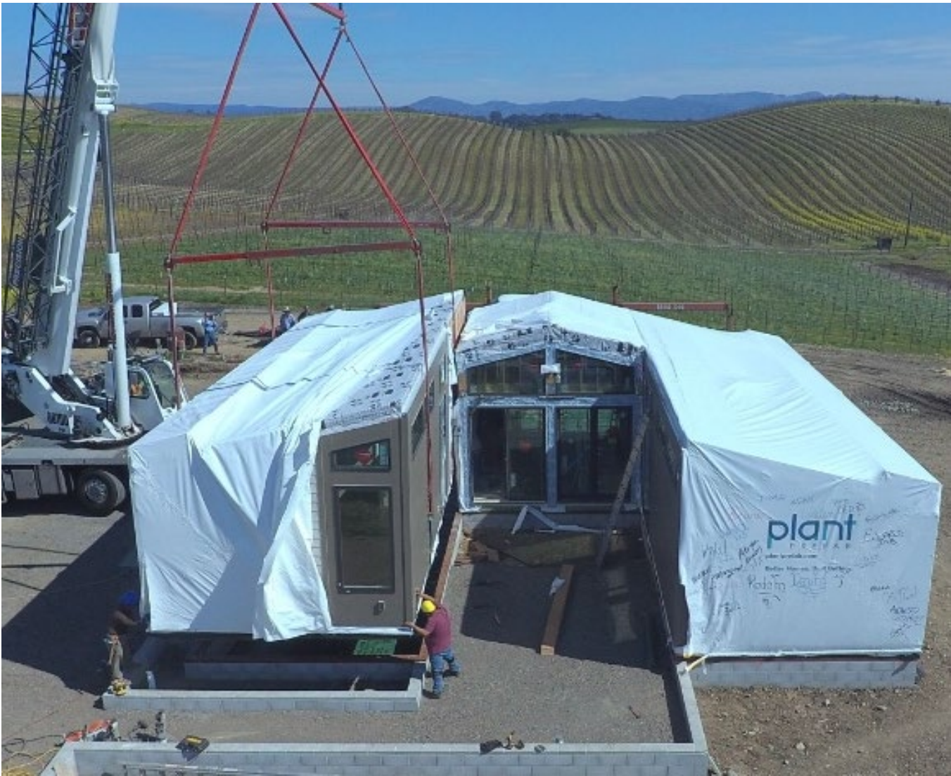
Modules are wrapped before departing the factory. On installation day (above), the hinged roof is visible beneath the plastic wrap, flipped up onto the main roof along the exterior walls.
