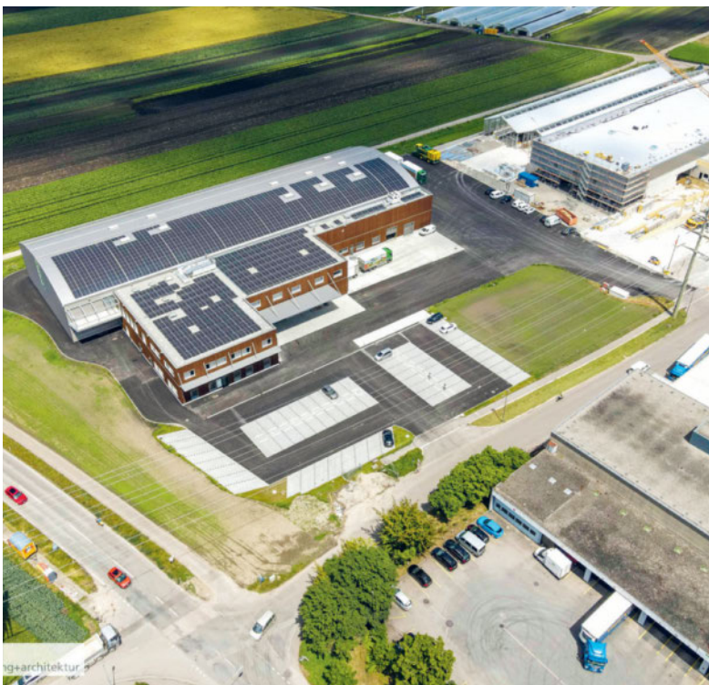
Photovoltaikanlage AHP Kerzers
