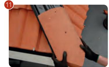
gaps at the eaves are covered. Remove the backing strip from the adhesive section and neatly dress onto the tiles. For optimal adhesion tiles should be clean and dry. Continue up the full length of the hip and over the ridge batten, overlapping each roll by at least 50mm.
