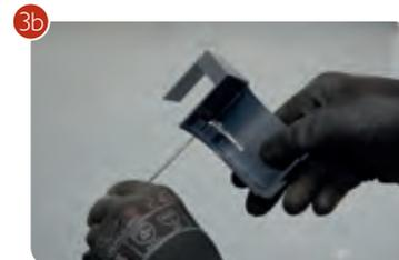
Using the nails provided in the Eaves/Ridge Pack, fix the eaves clip to the fascia board.
