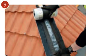
the tiles should not be more than 30mm from the hip batten. For Cambrian Slates: each cut slate (for type, see table below) must have at least two nails at the head and be clipped where possible.
