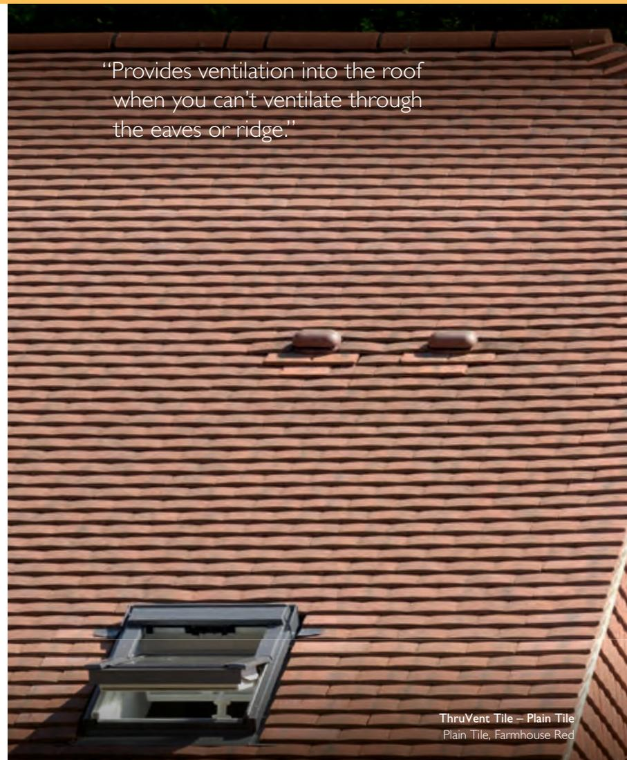
“Provides ventilation into the roof when you can’t ventilate through the eaves or ridge.”
