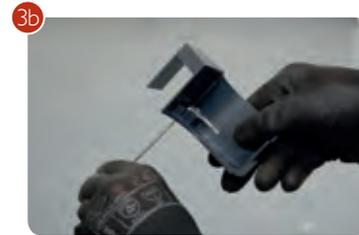
Using the nails provided in the Eaves/Ridge Pack, fix the eaves clip to the fascia board.
