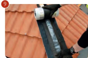
the tiles should not be more than 30mm from the hip batten. For Cambrian Slates: each cut slate (for type, see table below) must have at least two nails at the head and be clipped where possible.
