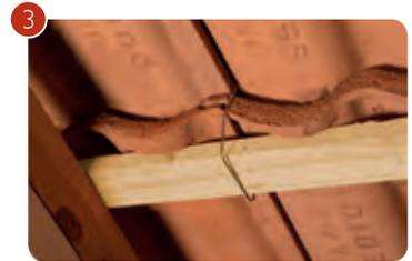
The Innofix Clip is installed by hooking onto the Redland tile interlock and then sliding beneath the 50 x 25mm roof batten, where it is then clipped into place:
