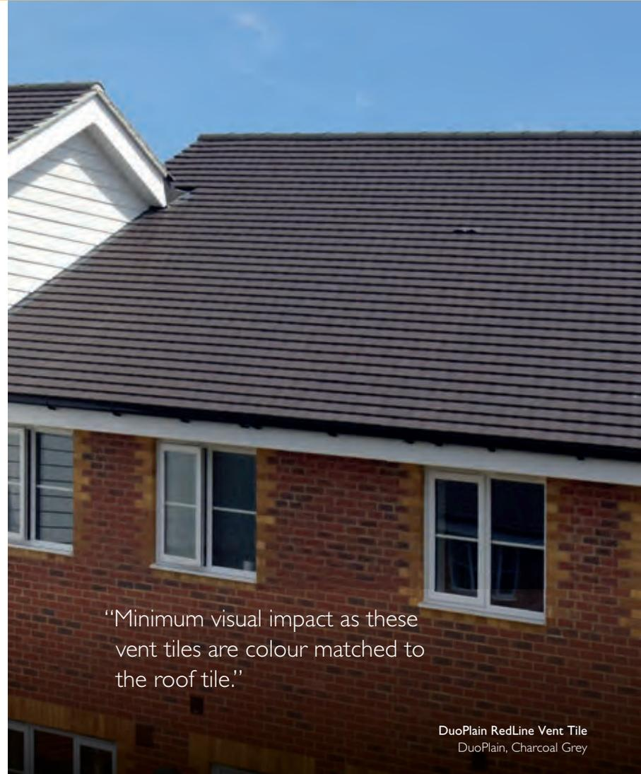
“Minimum visual impact as these vent tiles are colour matched to the roof tile.”
