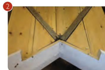
and nail fix into the rafters using 65mm batten nails, one per rafter.
